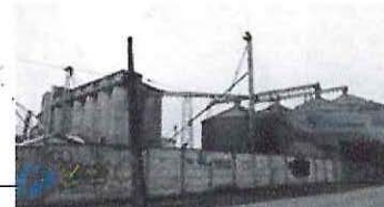
SILOS SAN FERNANDO
