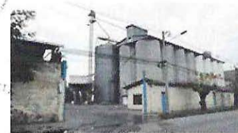
SILOS SAN FERNANDO
