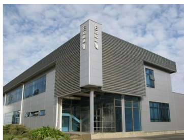
Figura 5: “Terminal Placilla, Valparaíso”
