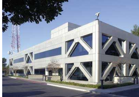
Figura 2.5. Fire Command and Control Facility Building
