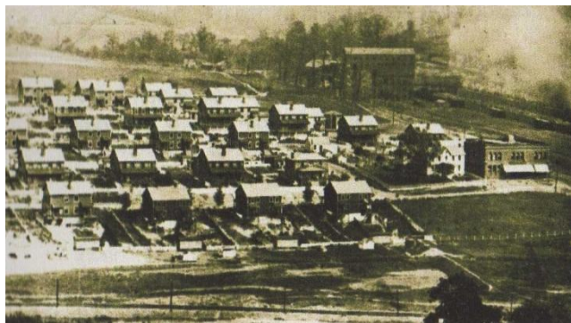
Shoaf, Georges Township, (Company Town) Fayette County, Pennsylvania
