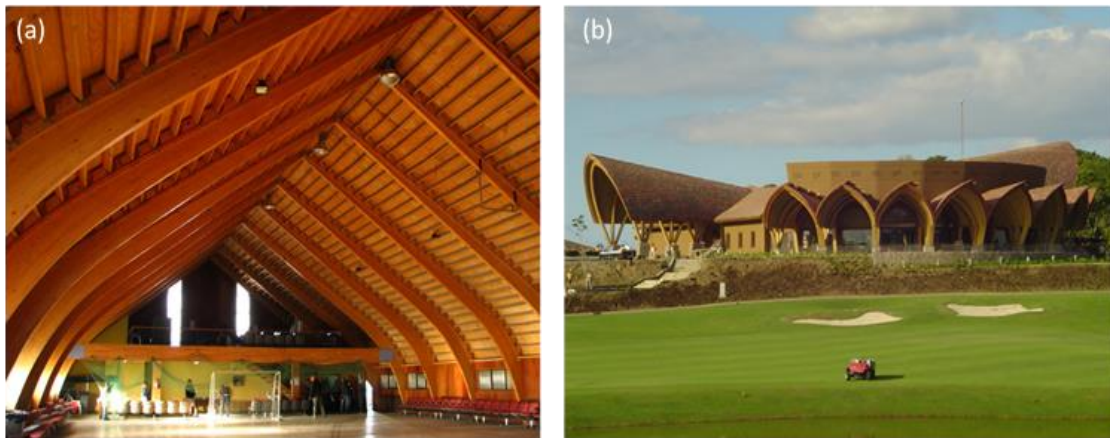
Figura 2.2 - (a) Gimnasio Valle Nevado, Chile. (b) Club de Golf Hotel Papagayo, Costa Rica [20].
